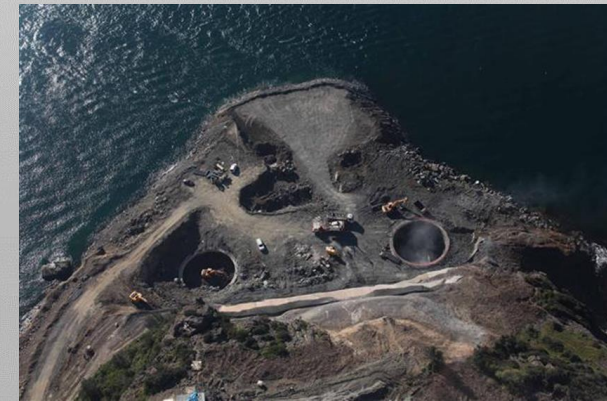
3rd Bridge Construction
